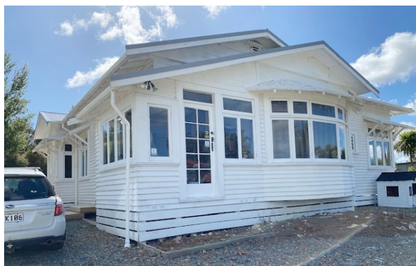
Here I am, sitting on nice new concrete piles
