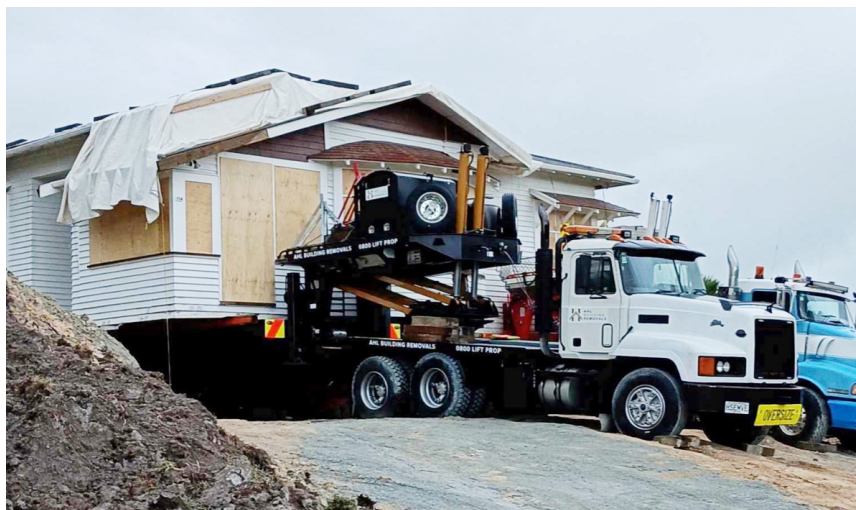
Backed up and I am together again; now I just have to get off the trucks
