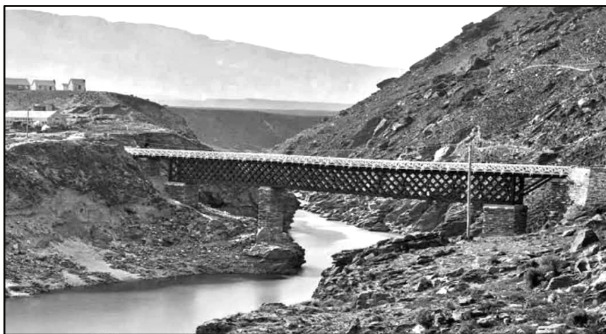
The wooden "lattice" bridge built in 1866 by the government
