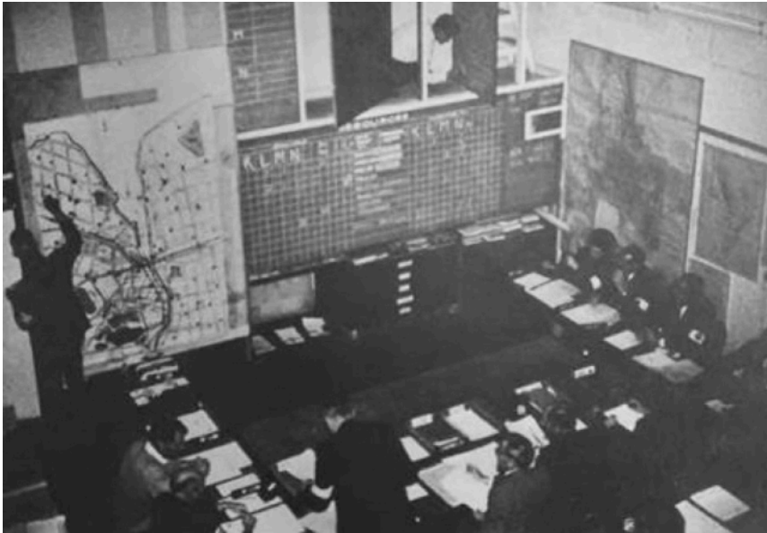
The former Filter Room reborn as the Civil Defence operations room
